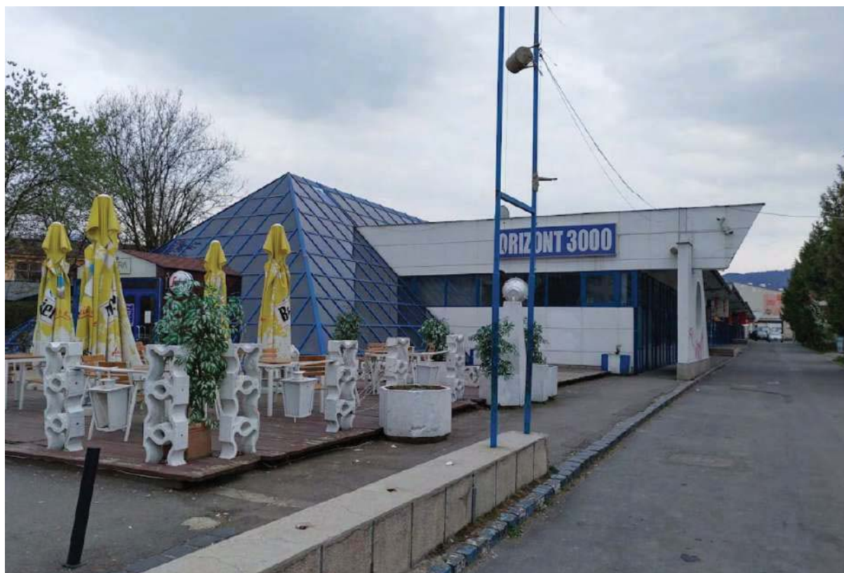
Fig. 51 - Complexul Comercial Orizont 3000
